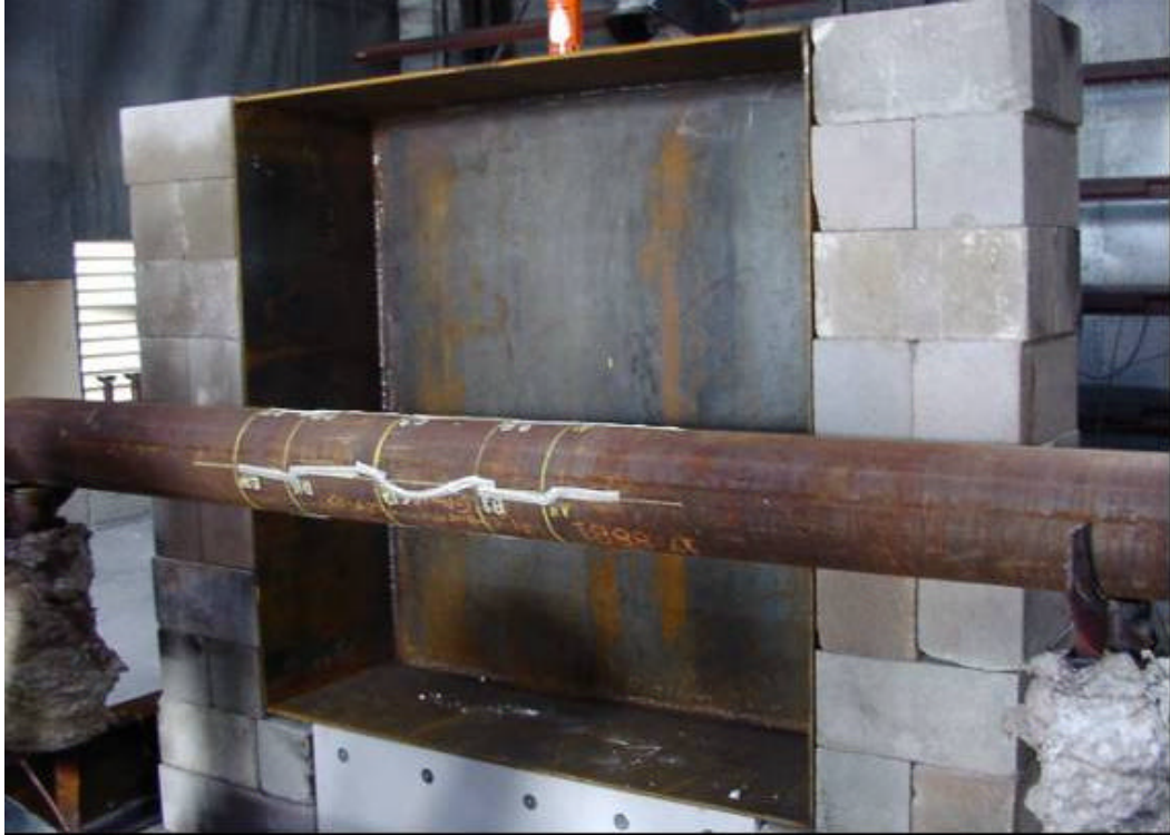
Figure C-1. Jet-Fire Tubular Section Prior to PFP Application.
